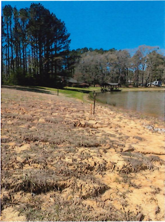
Lake level view of berm and trees to maintain
